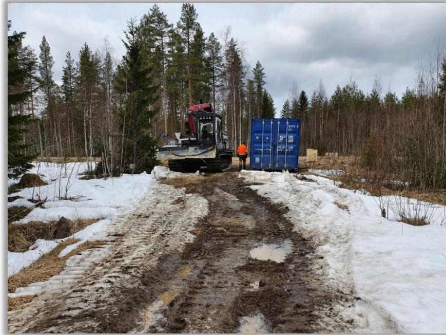
Figure 50 Drilling site 6 th May 2021 at Pontio.
